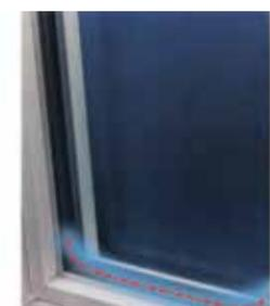
A dual seal, Warm Edge IGU featuring the Super Spacer® system is better able to ensure NFRC ENERGY STAR® certification by providing the best thermal conductivity, the lowest U-Value among dual-seal systems and the best durability available.
